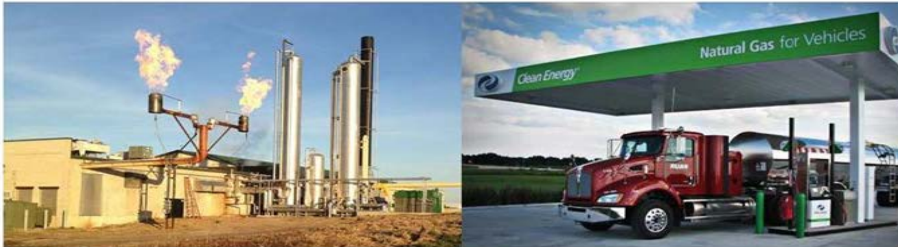
Fair Oaks Dairy Digester/Renewable Dairy Fuels
