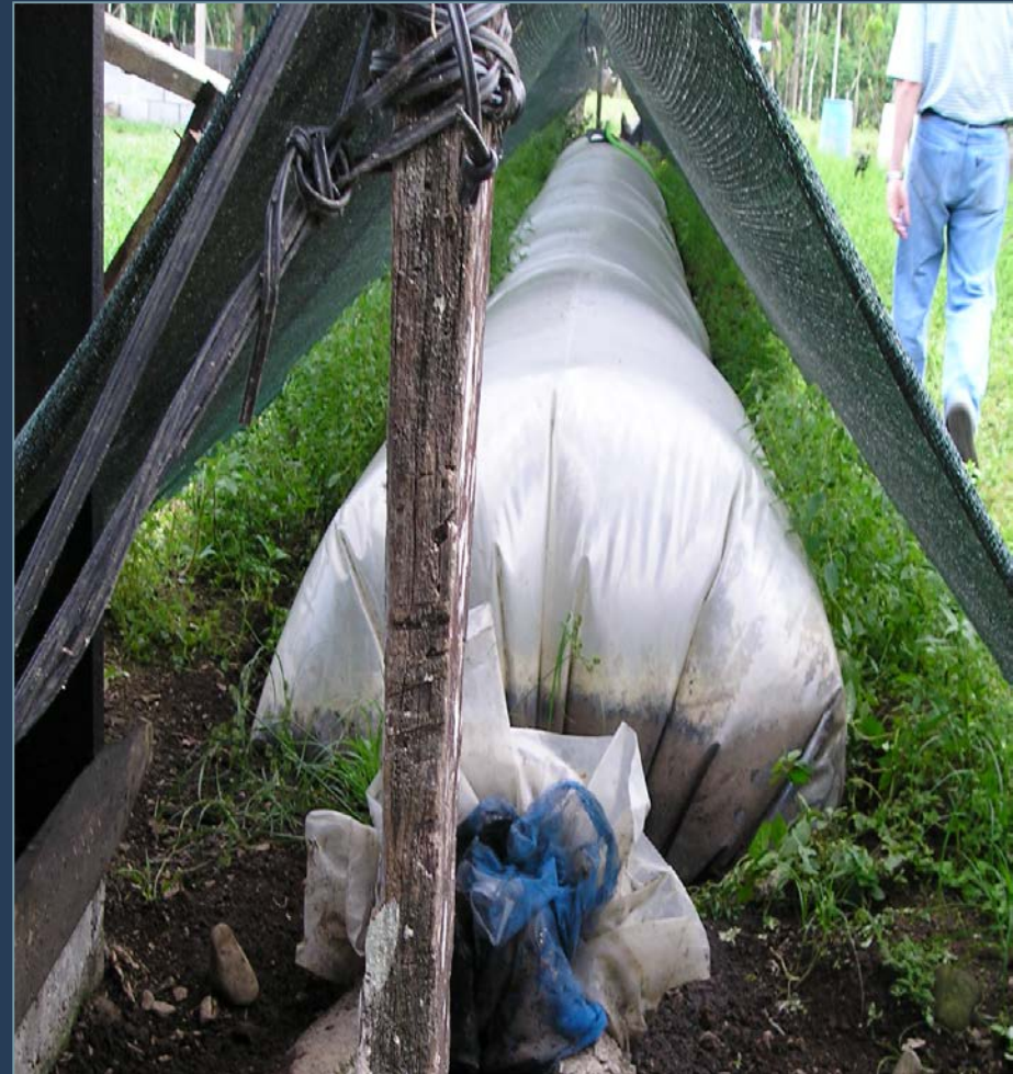
Dairy Manure Digester Guapiles, Costa Rica
